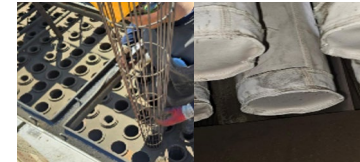
Replacement of Bag Filters for Dust Collectors
