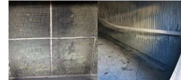
Catalyst Cleaning and Internal Repair for Denitrification Facilities
