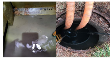
Dredging of Non-point Source (NPS) Pollution Control Facilities
