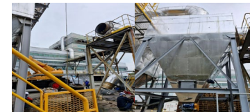
Replacement of Aging Dust Collectors
