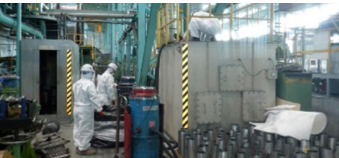
Replacing activated carbon in Adsorption tower
